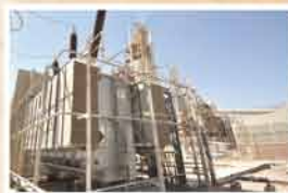
Power Transformers 32/40 MVA, 220/11 KV
